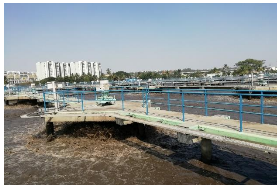
Mylasandra Sewage Treatment Plant
