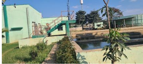
Kadubeesanahalli Sewage Treatment Plant
