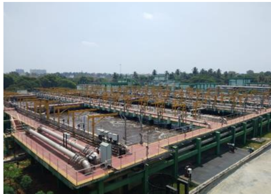
Doddabele Sewage Treatment Plant
