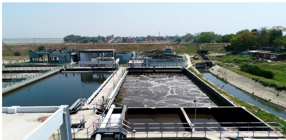
Sewage treatment using the SBR process
