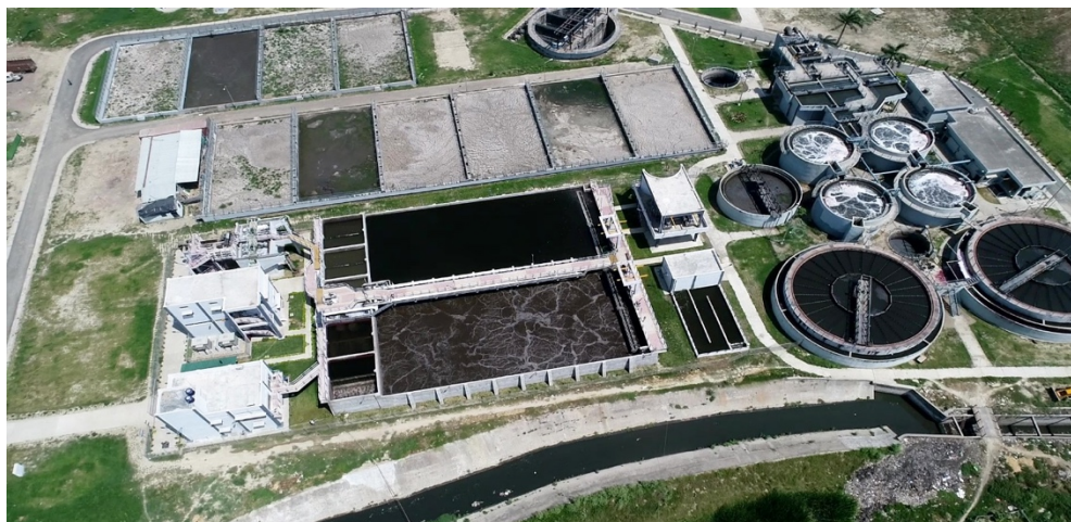
Full view of the Salori Sewage Treatment Plan (including the existing facilities)
